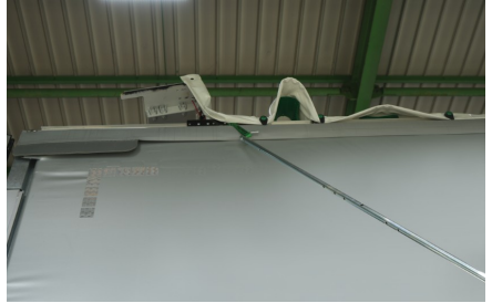
Sliding roof from outside
